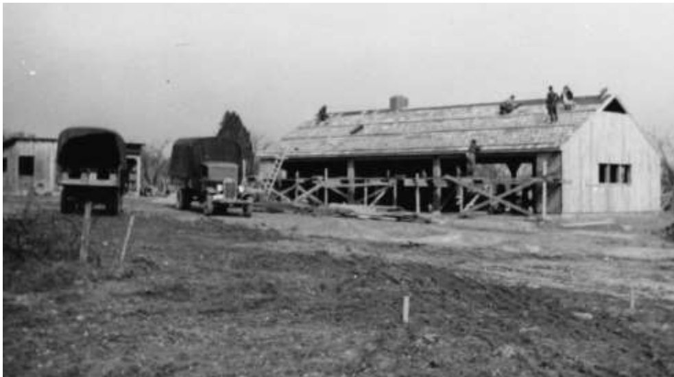
Construction of new storage building to replace old Hance barn, 1942.
