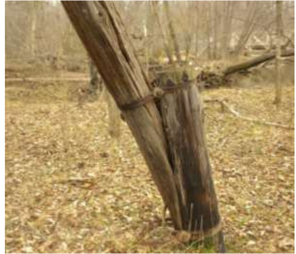
Old telegraph pole made of American chestnut wood near Duvall Bridge.
