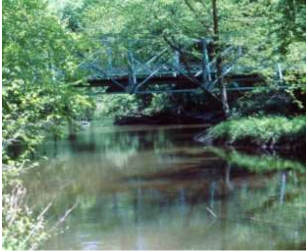
.Duvall Bridge over the Patuxent River
