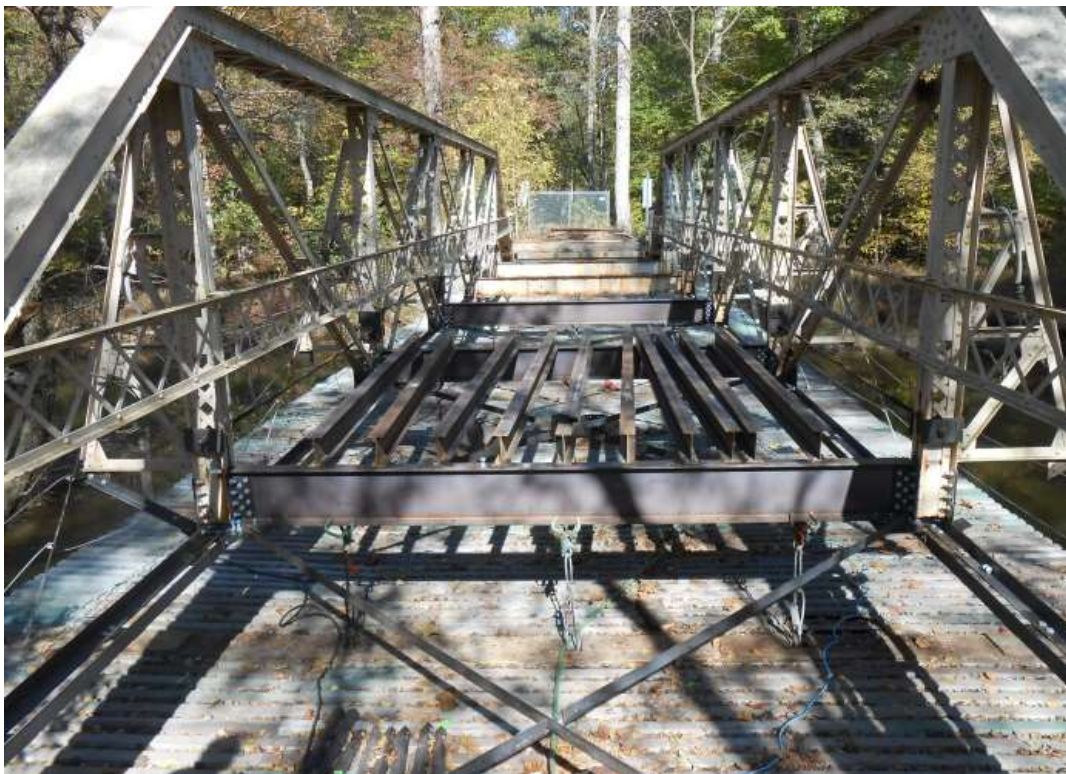
Duvall Bridge during restoration in 2015.
