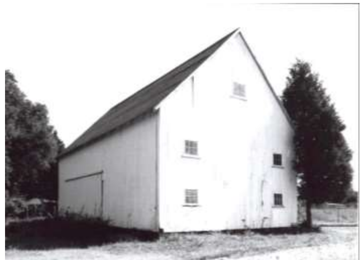
Lower Duvall Tobacco Barn, restored by WPA in 1930s. Photo by National Park Service, 1987.
