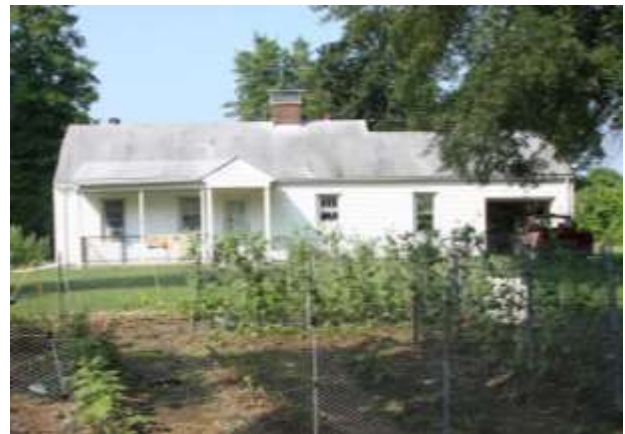
Back of Caretaker's House, 1980s.
